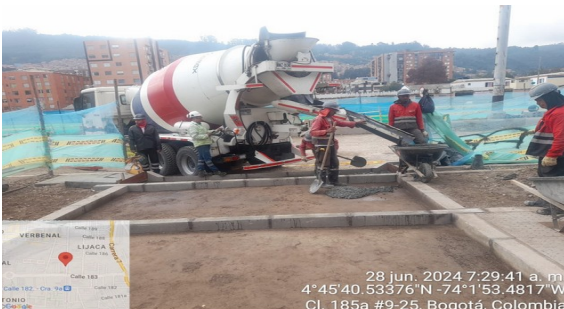
Fundida entrada Vehicular K1+440.
