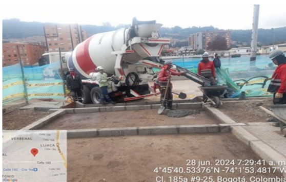
Fundida entrada Vehicular K1+440
